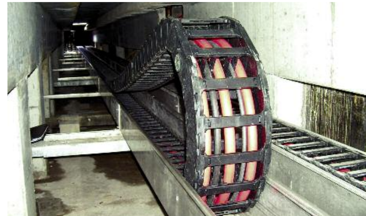
chainflex® CFCRANE for 500 m and more of travel. e-chain®: igus® rol e-chain®
